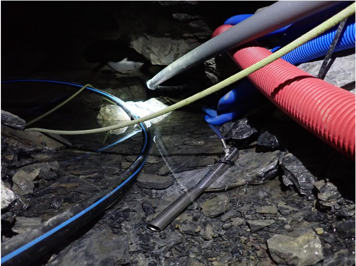
Appendix 5: p&T logger installed in the entrance of the Chlus cave in March 2023.
