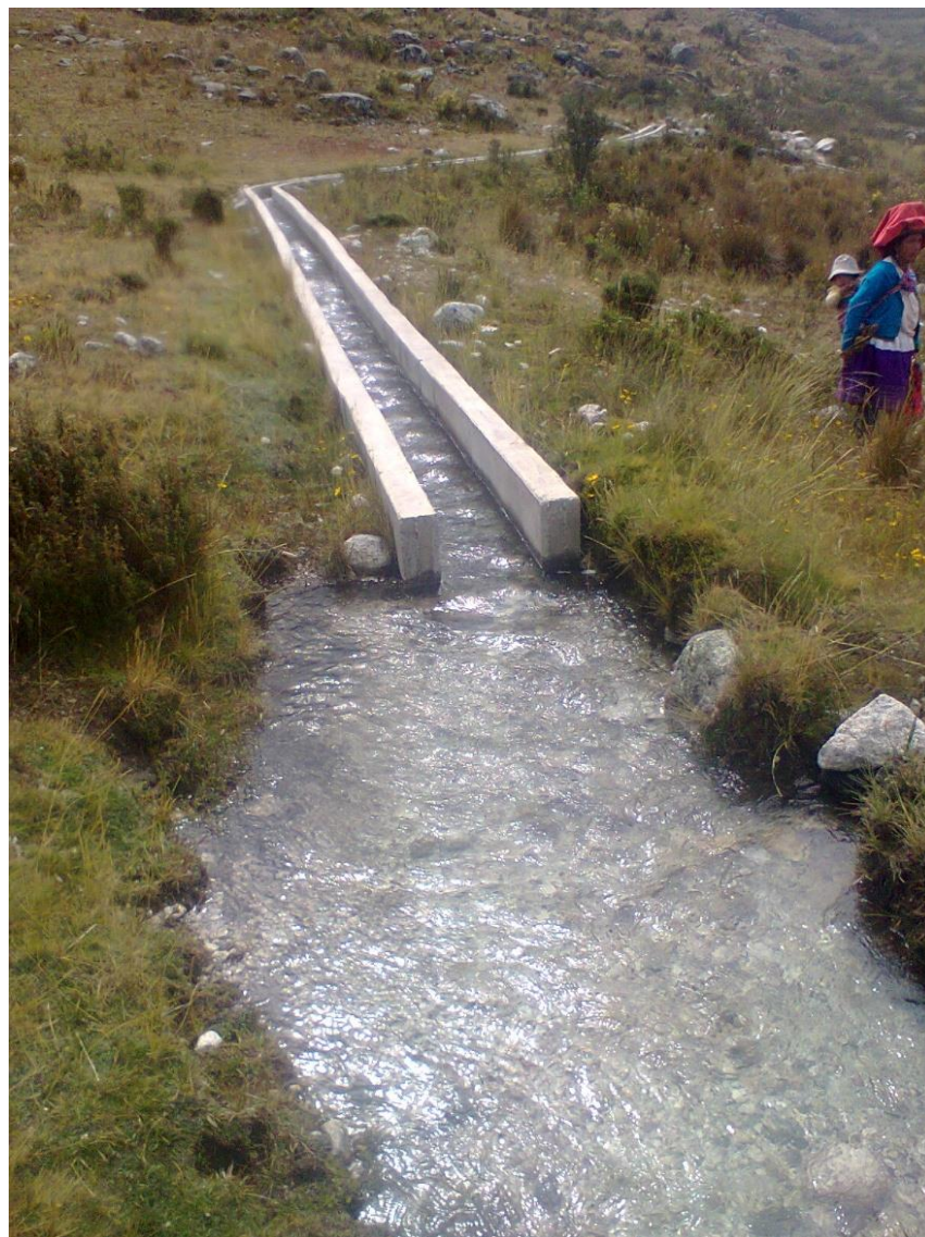
Figure 4. Irrigation water canal collecting water from natural streams and conducting it to the agricultural fields (Image retrieved from MINAM, 2014).
