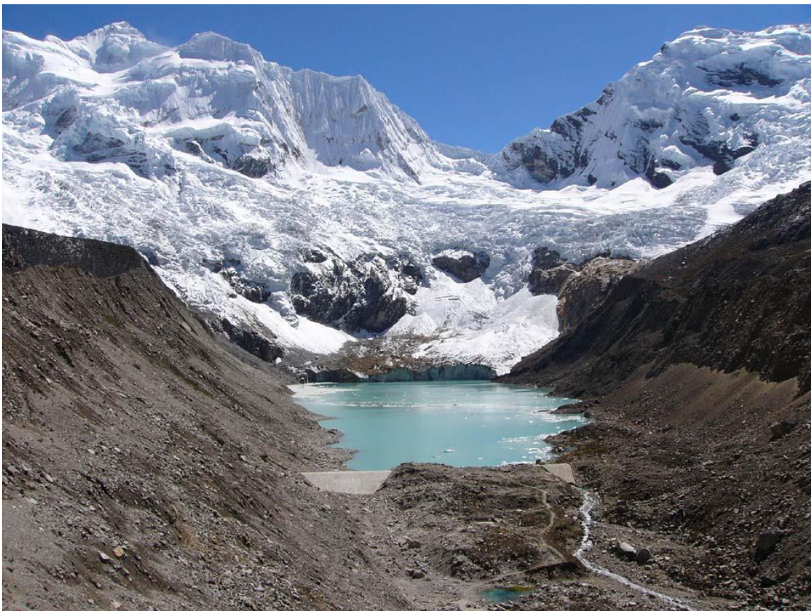
Figure 1. Lake Palcacocha in the North-Eastern part of the catchment, with its artificial dam stabilizing the lake outflow area (Picture retrieved from Zdenek Patzelt, 2004 in Vilimek et al., 2005).
