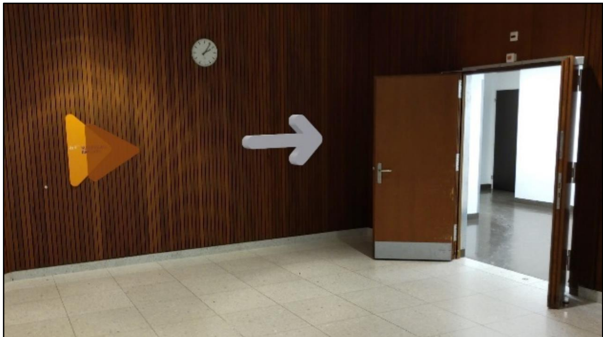
Figure 85: Intersection 2 at Y04-F-30.
