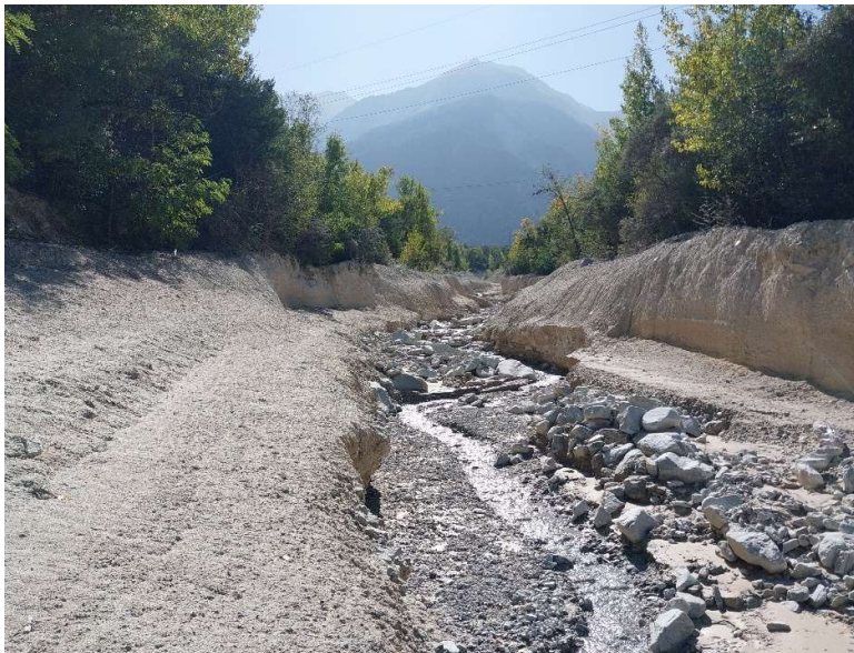
Figure 7: View of the channel above CD 28 on the day of the infiltrometer measurements. The mud caps can be seen on both sides of the channel. The measured mud cap is the one on the left of the image, so on the right in flow direction
