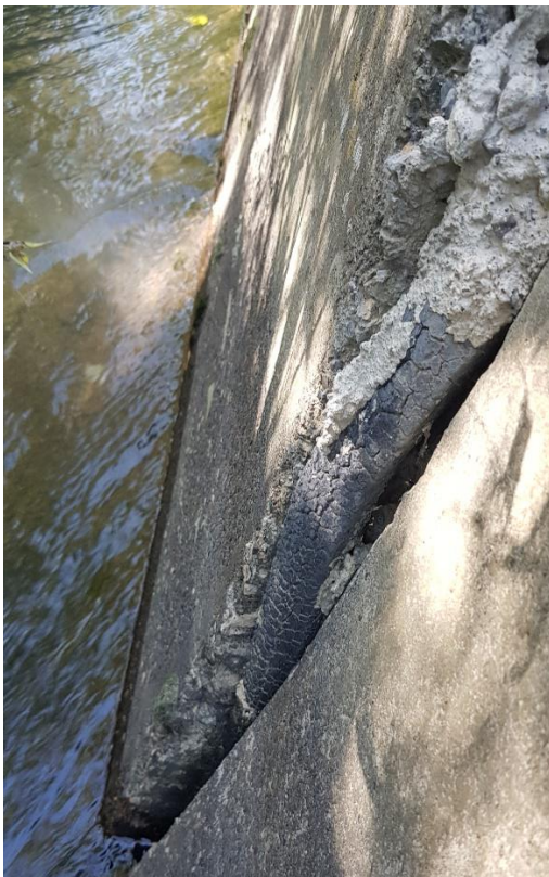
Figure 19: left shows old sealing of canals of the RWMD in Teploklyuchenka. Picture taken by Author, 6.10.2023
