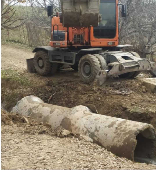
Left Figure 9: A ready-made latok on research site. Picture was taken by the author
