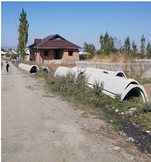
Figure 17: Latoks ready to install in Kyrgyz-Ata. Supported by Fundings of KOICA. Picture taken by Author, 6.10.2023
