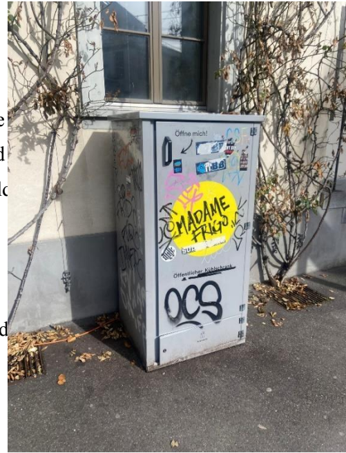
Figure 9: Frigo “Kalkbreite”, City of Zürich (Photo by Anja Schenk, 21.02.2024).
