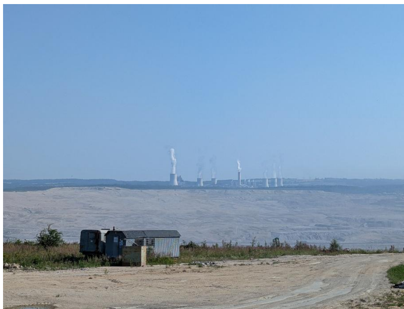
Fig. 12: Turów coal mine and power plant (own photo)
