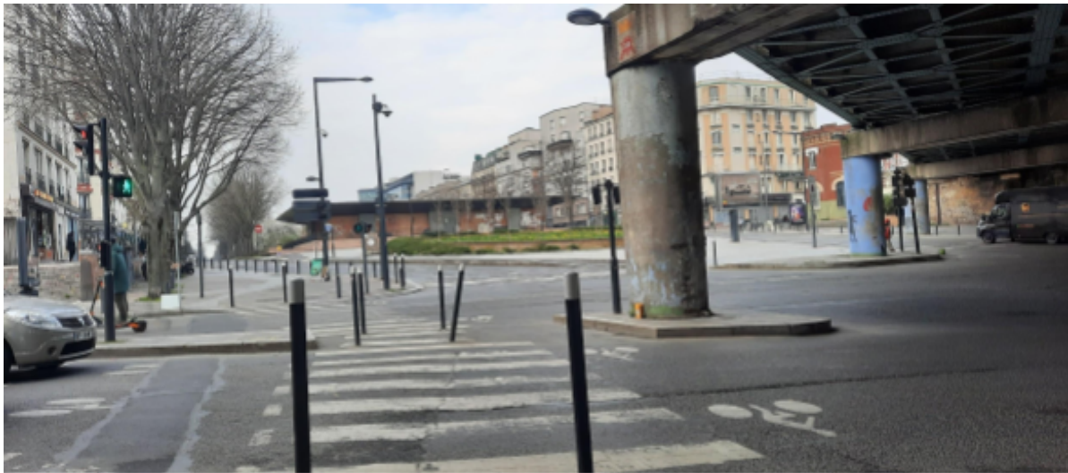
Fig. 7: Crossing at Rue du Landy, where the A1 motorway has been covered and transformed into a new boulevard (Author, 2025)
