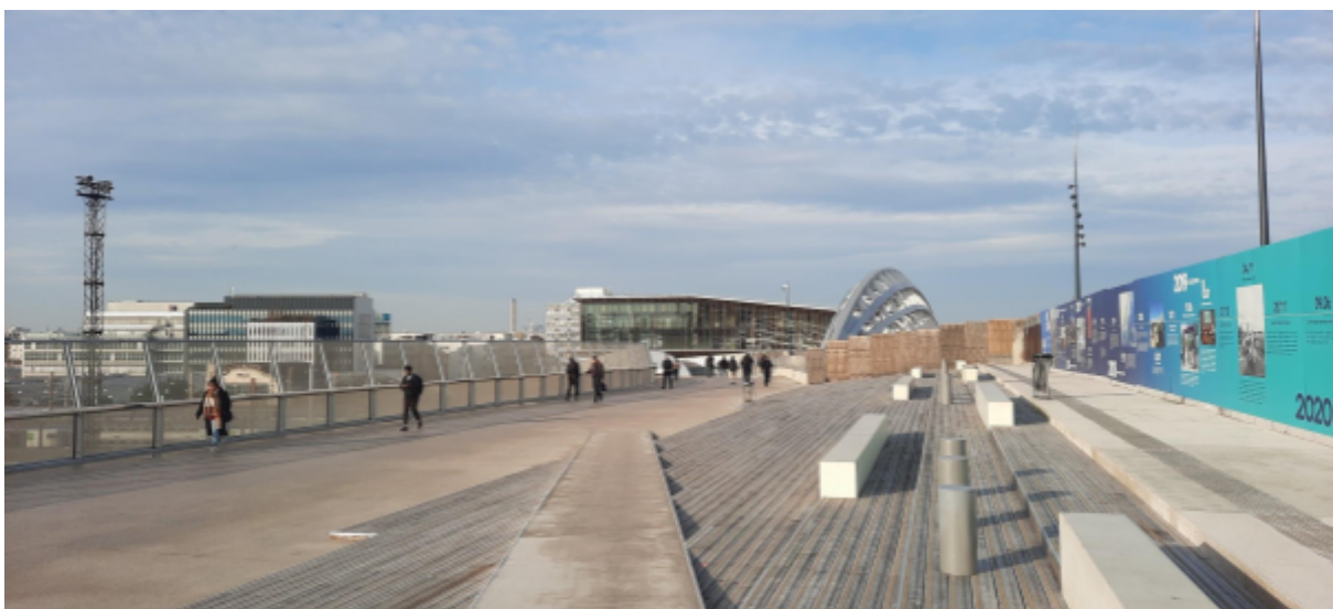
Fig. 8: Franchissement Urbain Pleyel (FUP) linking Pleyel and La Plaine constructed for the Olympics (Author, 2025)
