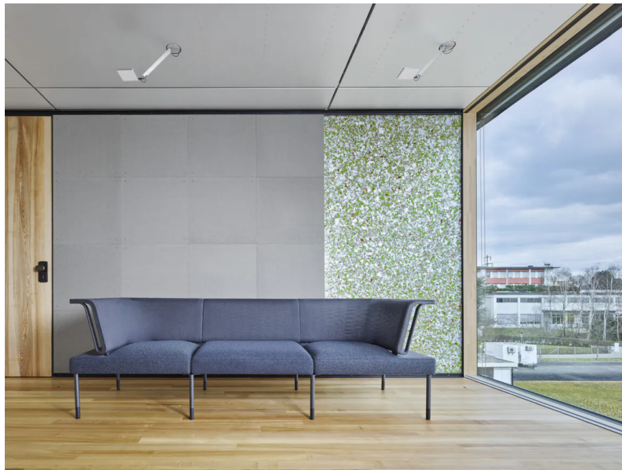
Figure 6: UMAR unit, showing innovative wall materials (e.g., Tetra Pak) (Braun, 2018).
