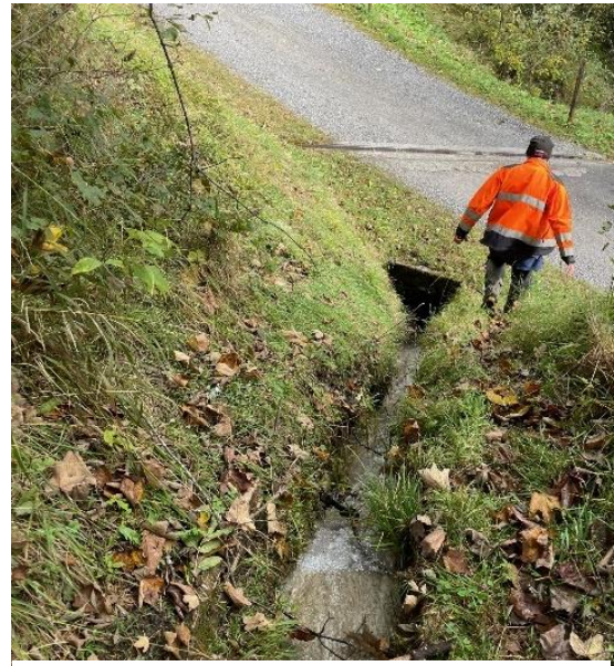
Figure 6: Inspection of individual drainage channels with the Elm forest ranger.
