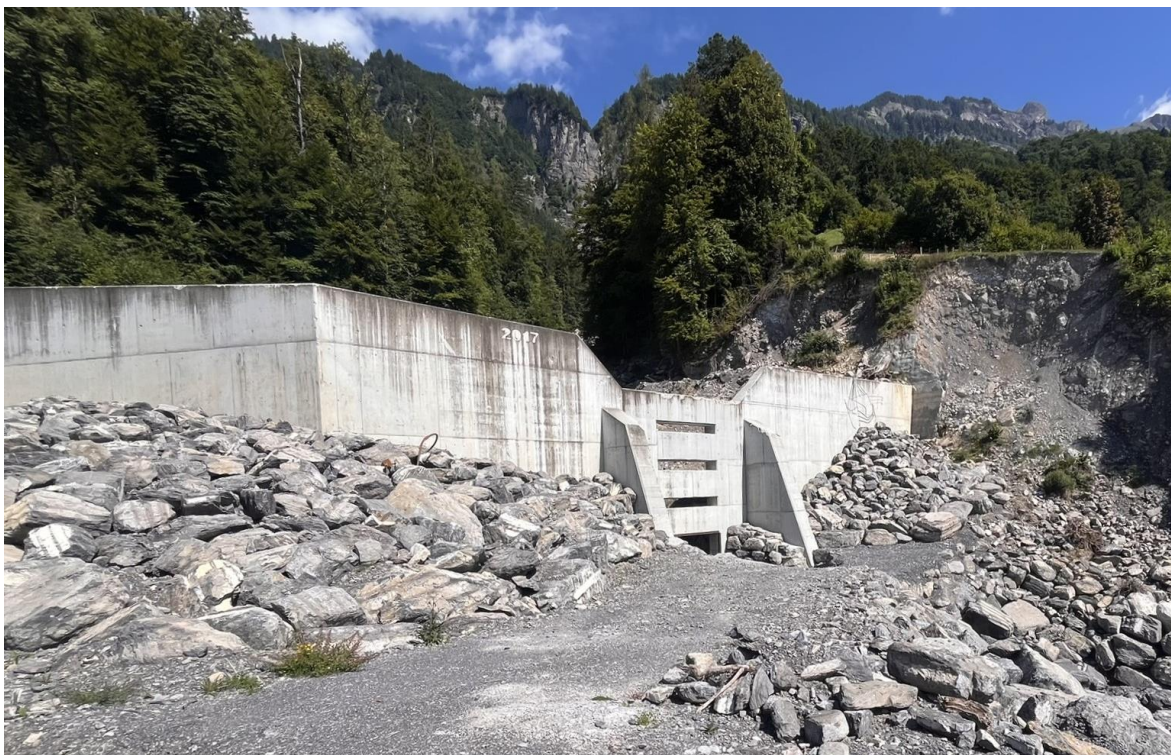
Figure 40 The retention wall in Brienz with a slanted and stepped crest to control the direction of overflow.
