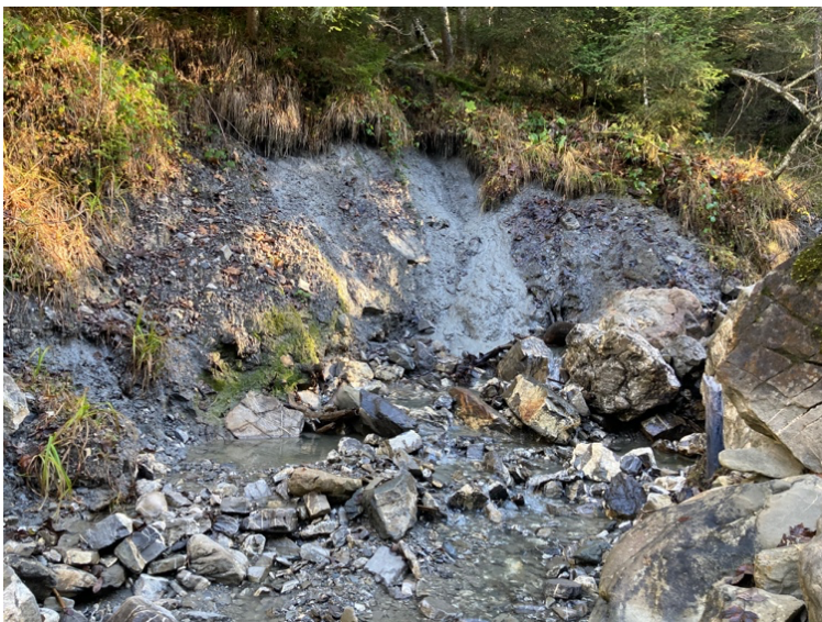
Figure 28. Active riverbank erosion at location S4 (Source: own photograph).
