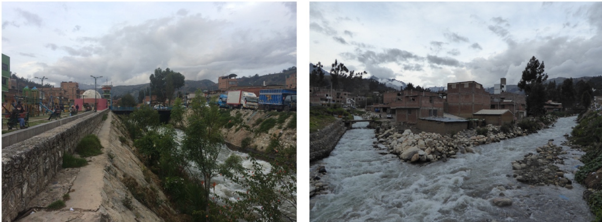
Figure 7 Infrastructure at GLOF risk. (left) Boulevard beside the Quillcay river in the city centre; (right) housing in the confluence of Paria and Auqui river in Nueva Florida. Source: photos by the author.
