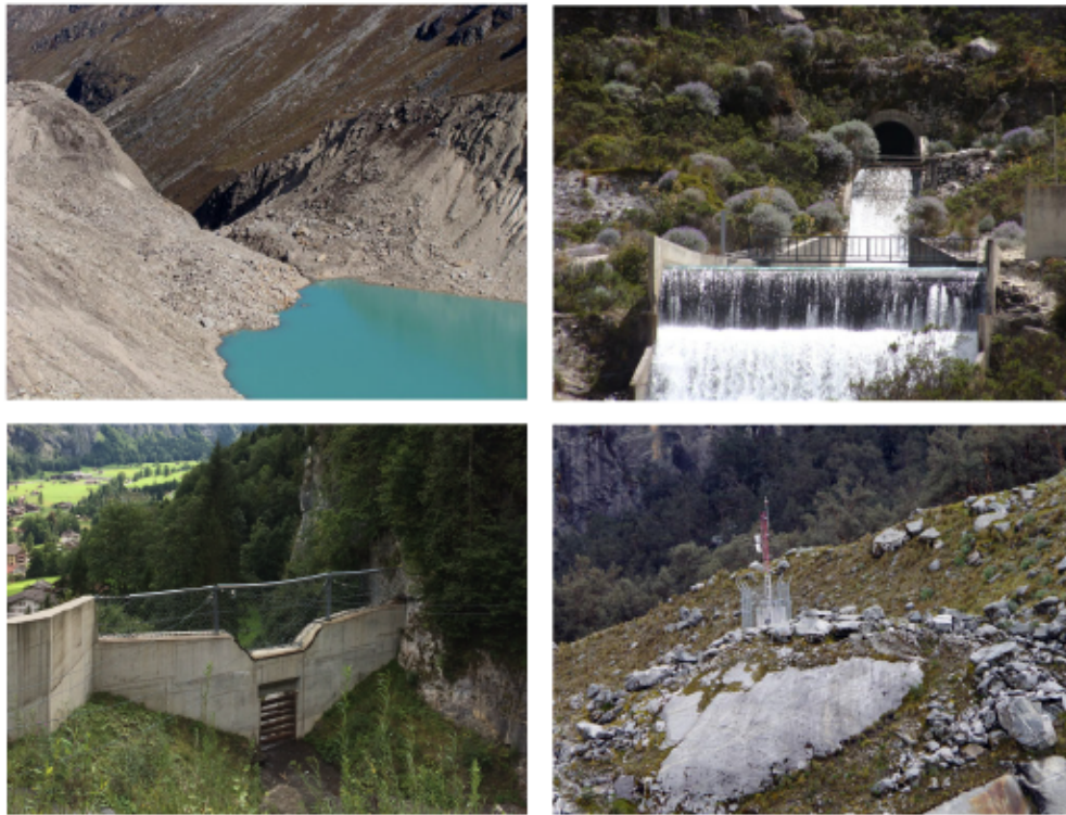
Figure 11 Examples of structural and non-structural GLOF measures. (top left) A failed moraine dam equipped with an open cut; (top right) an outlet of a drainage tunnel; (bottom left) a retention basin; and (bottom right) a transmission tower of an early warning system. Source: Emmer et al. (2018) except for the retention basin which is a photo by the author.
