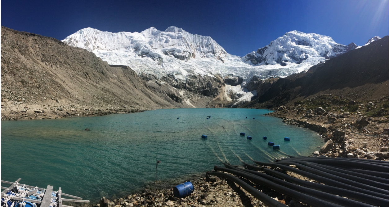
Figure 5 The Palcacocha glacial lake. The two glaciated mountains Palcaraju and Pucaranra are located in the background. In the foreground the siphoning system which drains the lake is visible. Source: photo by the author.
