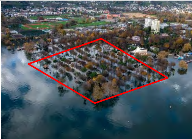
Aerial image - 16 November 2014
