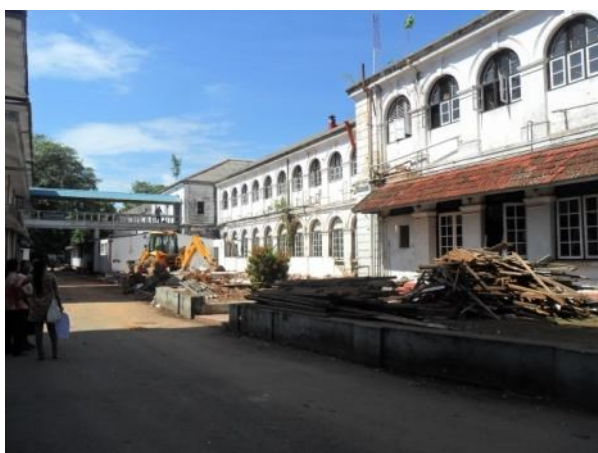
Figure 8: Auditor General's Department Building before reconstruction (Source: UDA, 2014)
