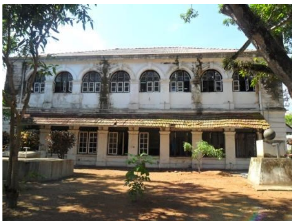
Figure 6: The building was overgrown before reconstruction (Source: UDA, 2014)
