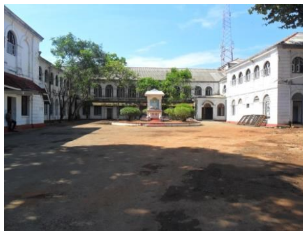
Figure 7: The outside courtyard before reconstruction (Source: UDA, 2014)
