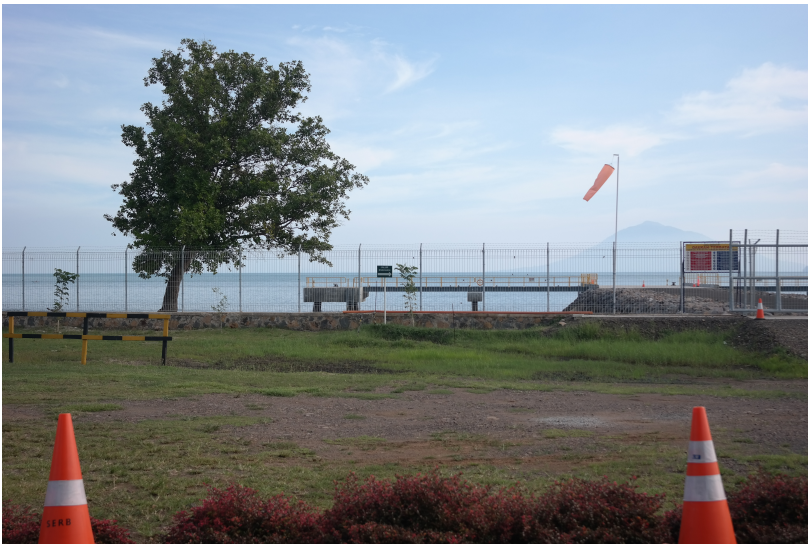
Figure 8: Supreme Energy's jetty at Sukaraja village (author, 2016)
