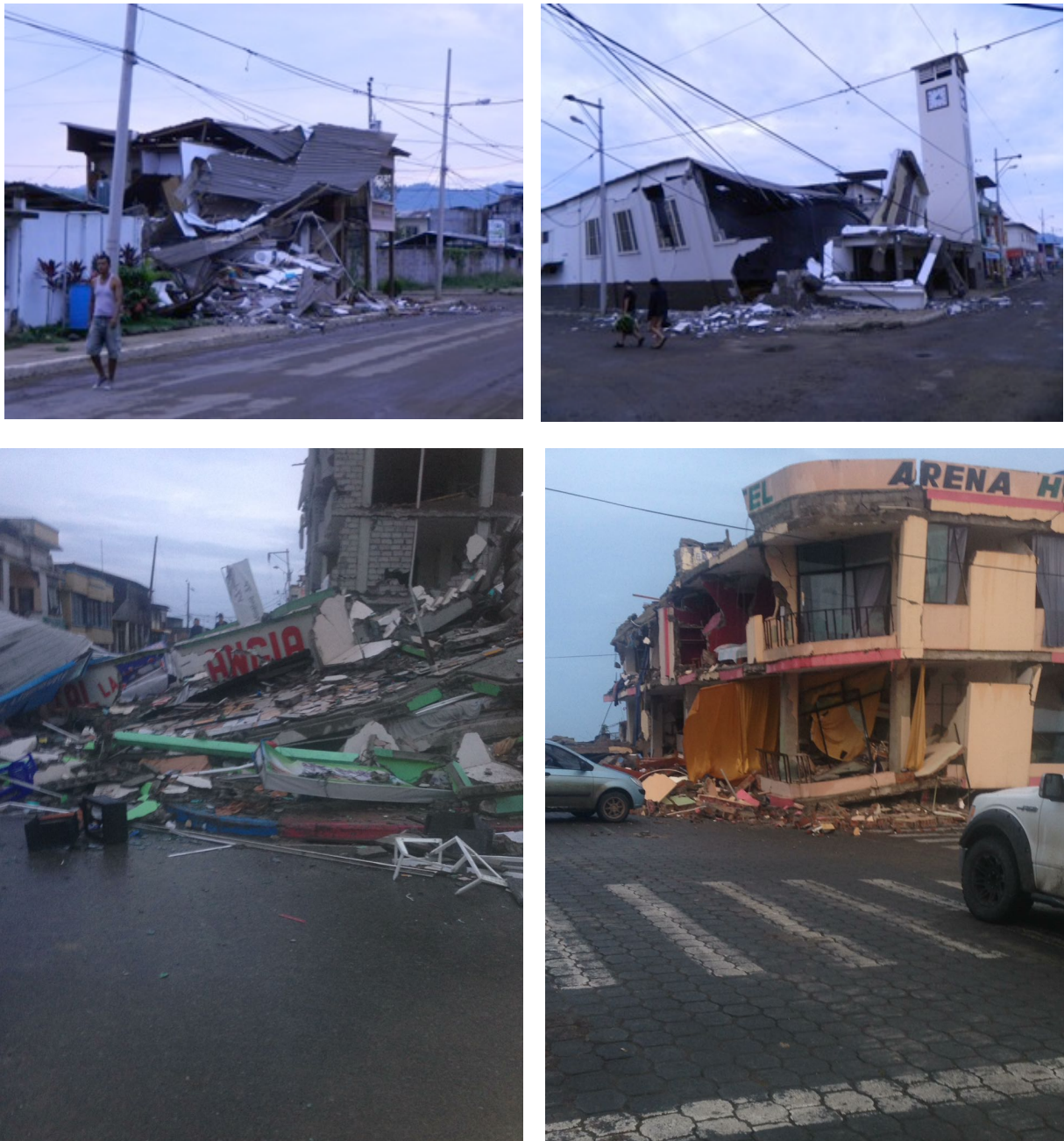
Picture 2: Destruction of the 2016 earthquake. Upper two pictures: Jama, Ecuador (Source: Photography by Xavier Cevallos, Jama, Ecuador); Lower two pictures: Pedernales, Ecuador (Source: Photography by Jorge, Pedernales, Ecuador)
