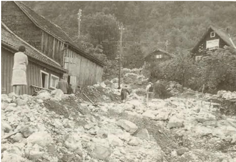
Figure 1: Deposition of the debris flow in Lienz on the 3 rd of July 1967 (Meier und Partner AG, 2017).
