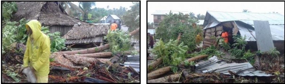
Damage from Cyclone Mona: Arorae, Kiribati 2019 (source: Onorio)
