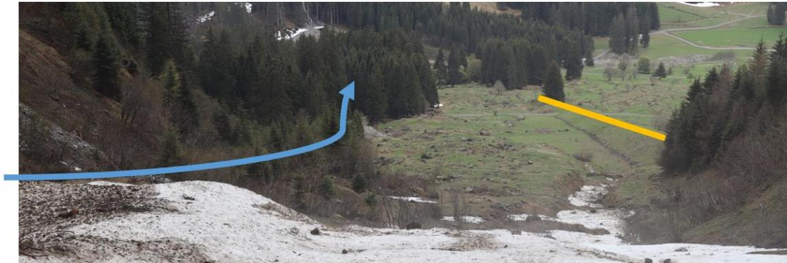
Figure 21: Situation when looking down from the fan apex at the Fraschmardin torrent. The location of the actual channel is marked in blueish colour, while the protection dam is coloured in a yellowish colour.
