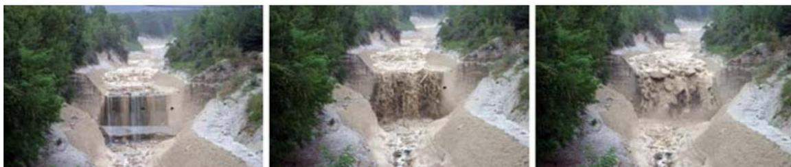
Figure 20: Arrival of the debris-flow front upstream of check dam 29 during the July 28, 2006 event (C. Gwerder, WSL). (Badoux *et al.*, 2009)
