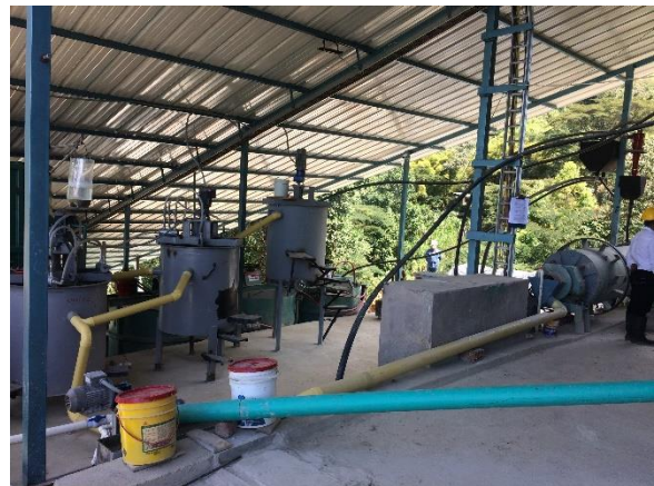
Figure 2: Processing plant next to some mines of ASMO 1 (Source: own photo).
