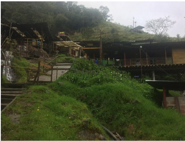
Figure 3: ASMO 2 infrastructure: processing plant on the left, entrance to the mine behind it (Source: own photo).
