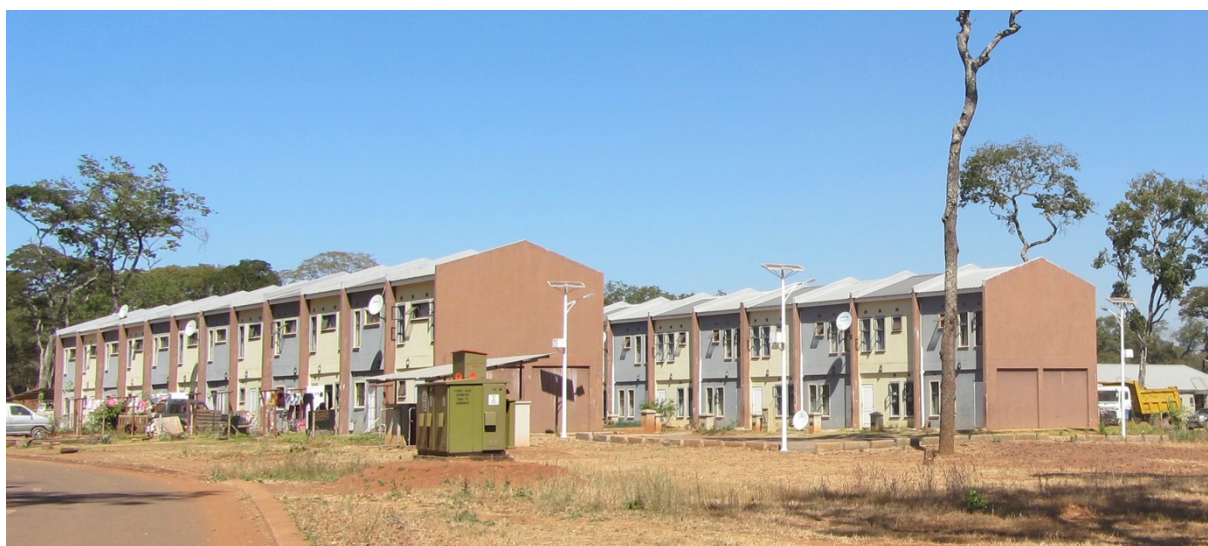
Figure 13: Two-Storey Terraced Houses in Kalumbila (own photo, 16.7.19)
