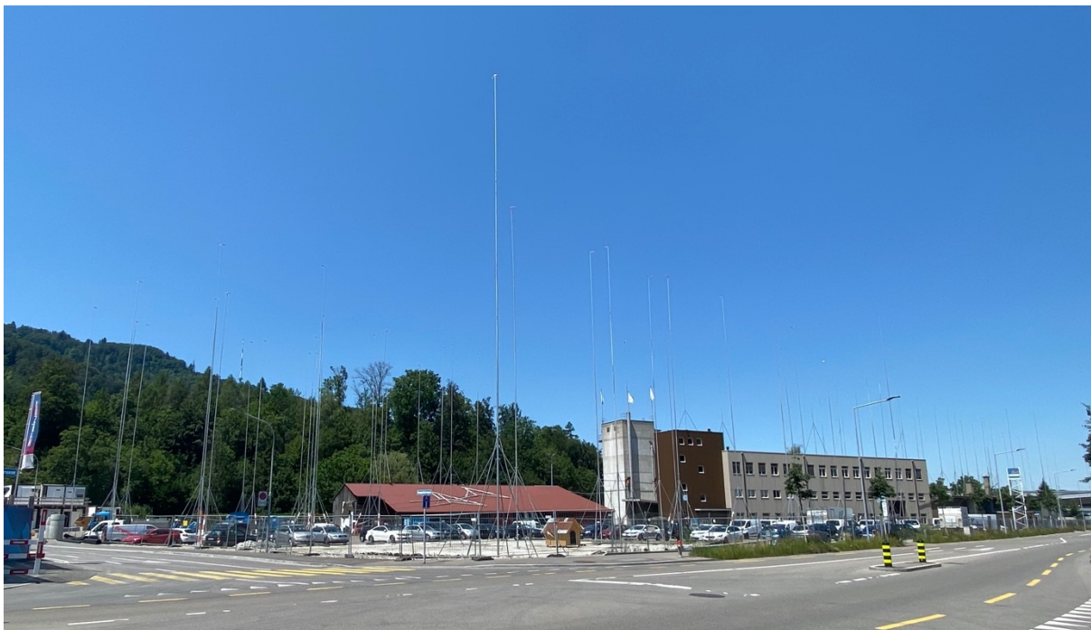
Figure 20: Construction spans staked out on Allmendstrasse 96 in Manegg, Switzerland.
