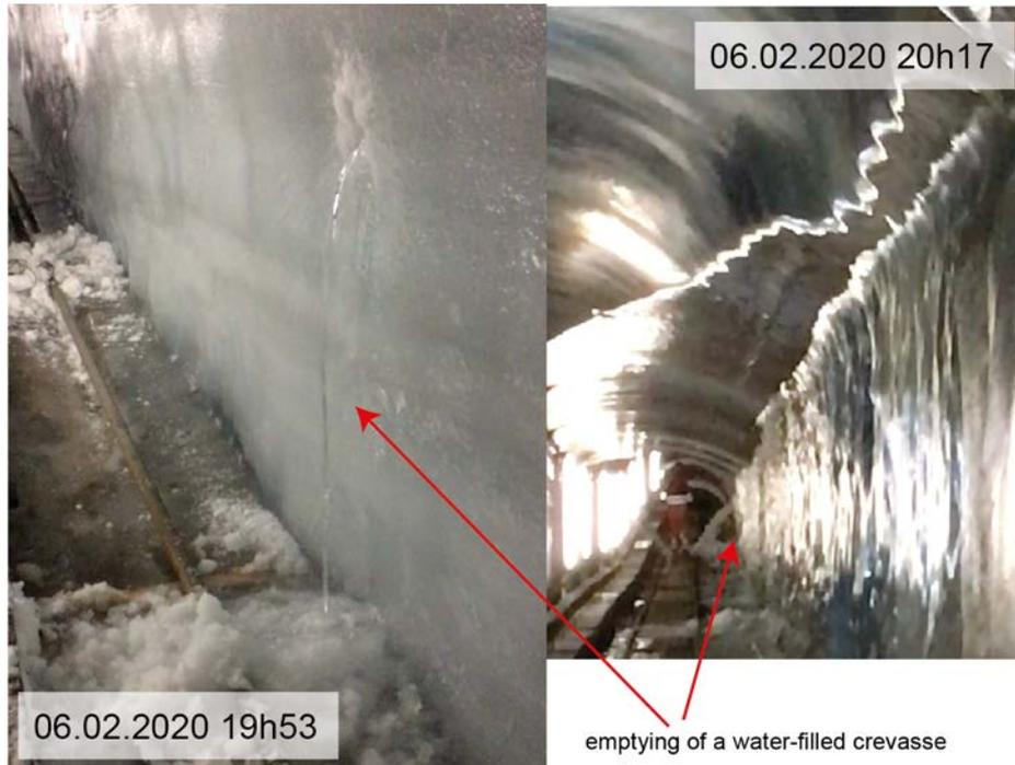
Figure B.2 – Emptying of a water-filled crevasse on 06.02.2020 (photo taken by S. Morard)
