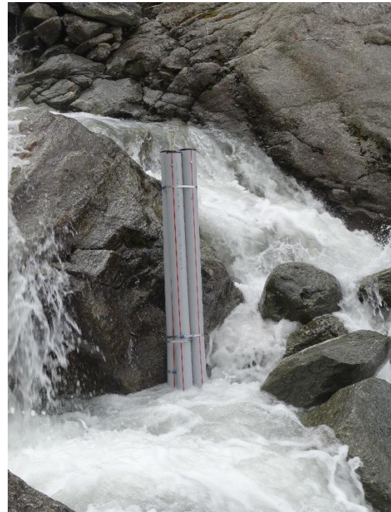
Figure 8: The installation of the stilling tubes in the Riedbach. All four tubes needed to be secured to one T-stake since it was impossible to drive more than one stake in the riverbed.
