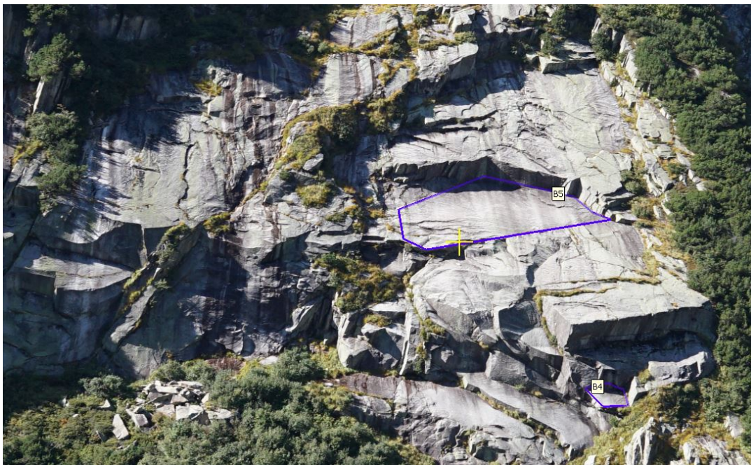
FIGURE 5.14: Handegg: Same area shown in Fig.5.13. Showing two failed blocks that were identified. They are limited with a violet polygon. There is a central one and the other is in the bottom left part of the picture.
