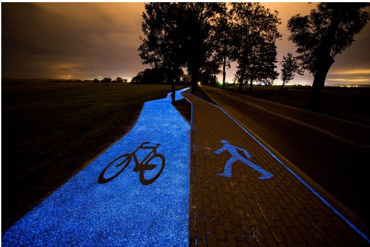
Figure 8: This bikepath is near Lidzbark Warmiński in Poland. It contains phosphors that are charged with sunlight during the day and then glow during the night (TPA Sp. Z oo, 2016).
