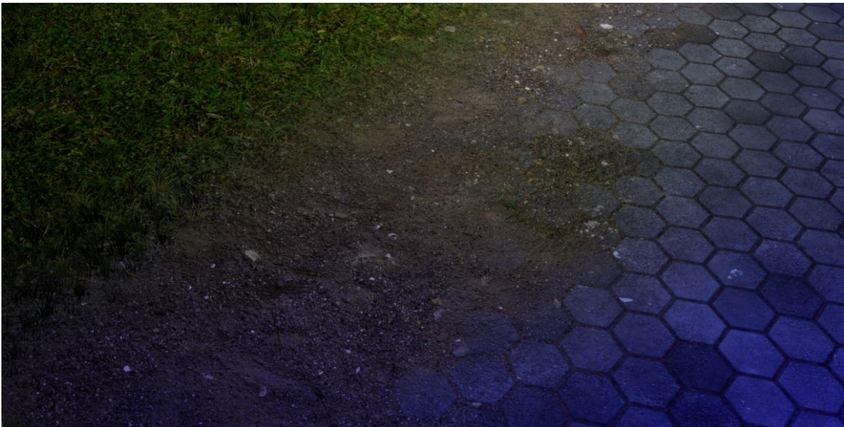
Figure 26: I tried to make the transition between road and lawn as smooth as possible.
