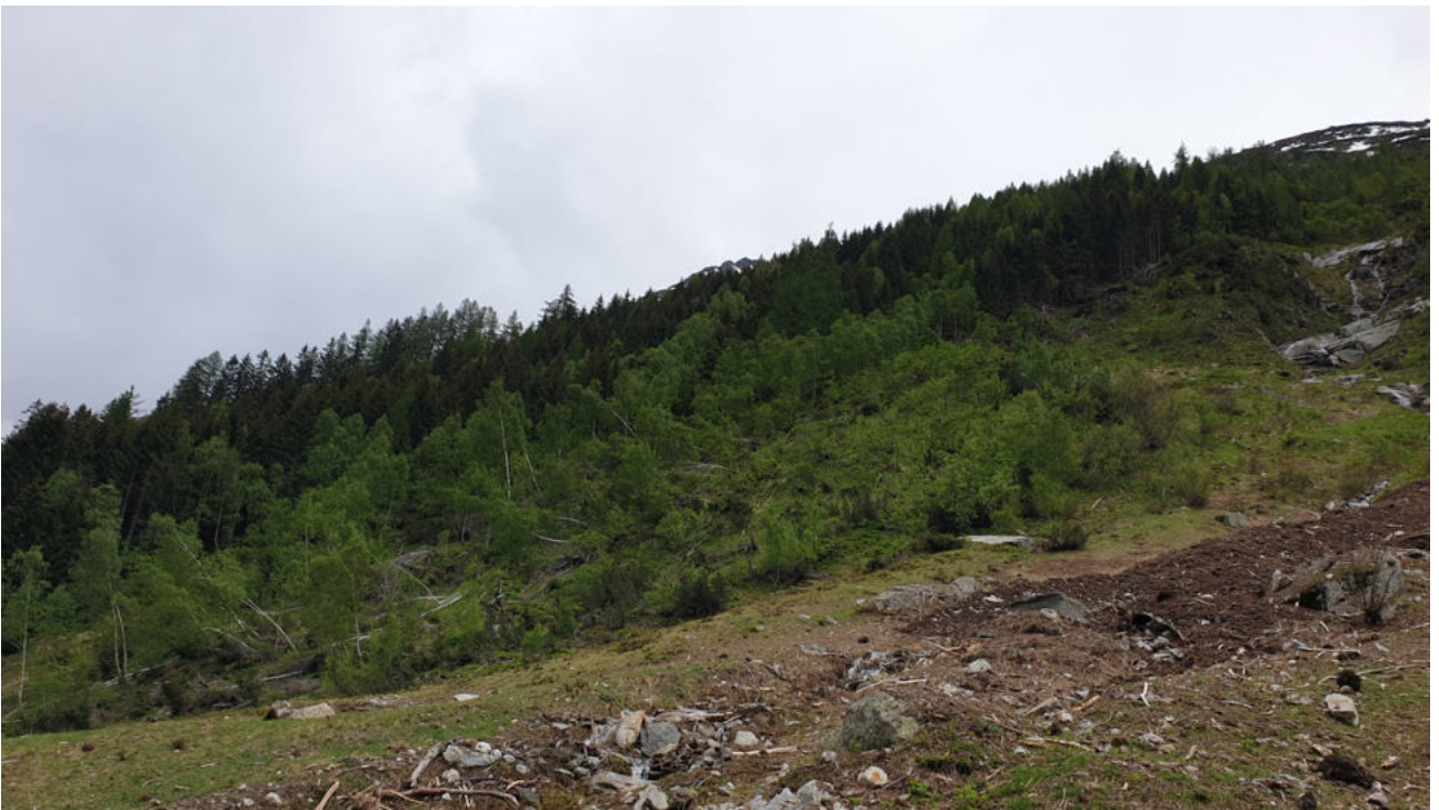
Figure 46: Pushed over and strongly bent trees on the eastern side of the study site.
