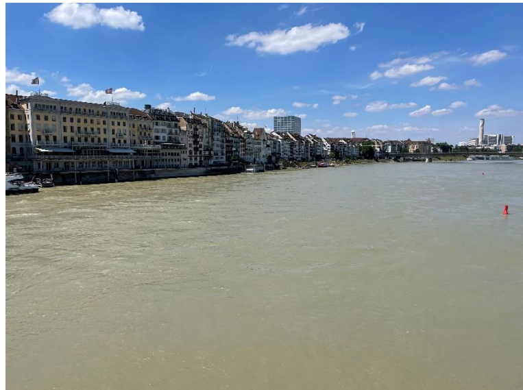
Figure 42: Row of houses along the Rhine which blocks cool air to enter the city (own image).
