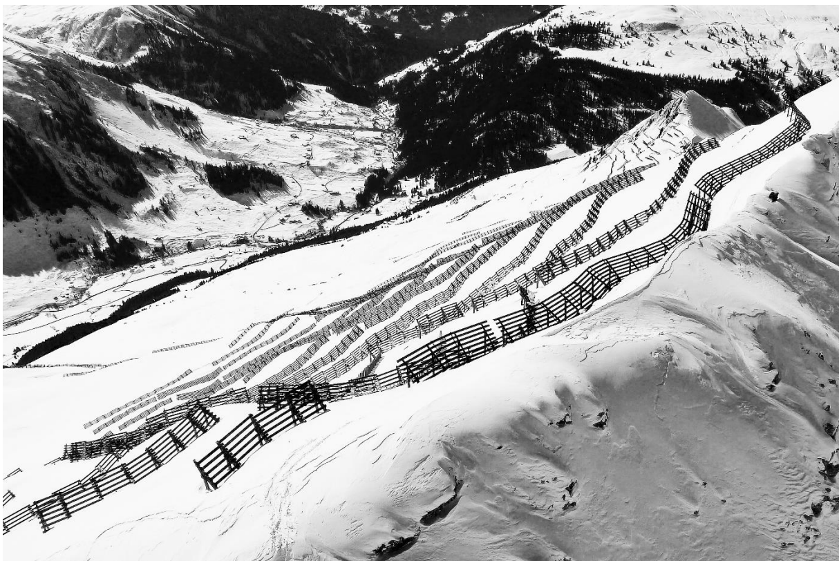
Fig. 5: The avalanche barriers on Chüenihorn with a view towards the St. Antönier valley. Source: Kaspar Thalmann.
