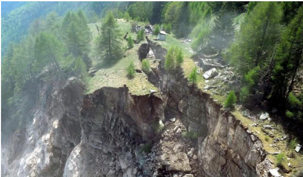
Fig. 8: The crevassed area above Preonzo TI: The part of the rock that has not (yet) been collapsed will continue to be monitored. Source: Geotest.
