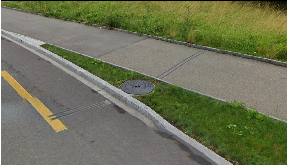
Figure 5: Example of an Induction Loop in Glatthbrugg (Screenshot of Google Street View on www.maps.google.com , accessed on 16/08/2023)
