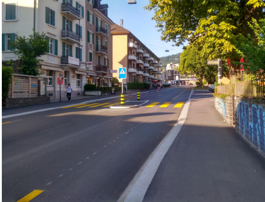
Figure 4.6: Interruption of bicycle lanes and road bottleneck due to pedestrian island. Source: bikeable.ch, user: lee_
