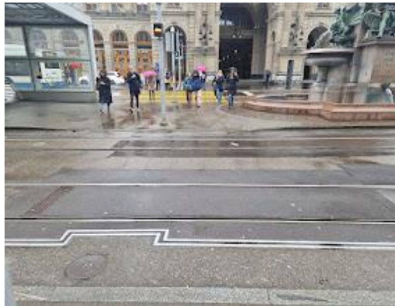
Figure 25: Incorrect curbs and difficulty of tram tracks (Picture by Silvia Juen).
