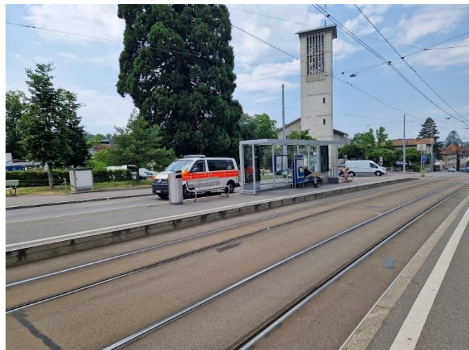
Figure 28: View of the Balgrist tram stop Without digital information sign and acoustic signalling option and entry marking for wheelchair users (Picture by Silvia Juen).
