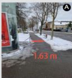
Figure A: Narrow pavement (red line), wheelchair users cannot pass one another
