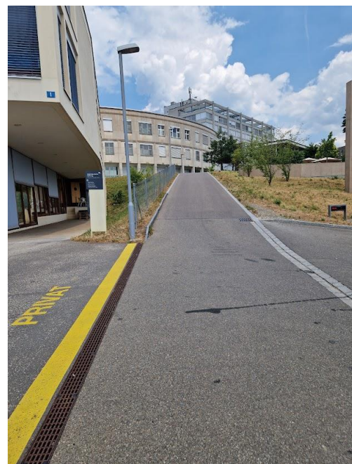
Figure 19: A standardized slope at the Mathilde Escher Heim, but without safety railings (Picture by Silvia Juen).
