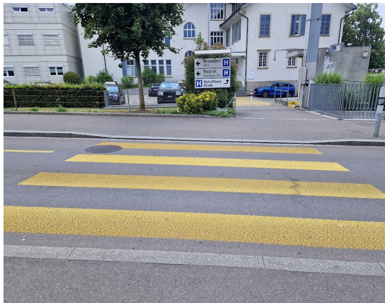
Figure 20: Example picture of non-standardized curb edge (Picture by Silvia Juen).
