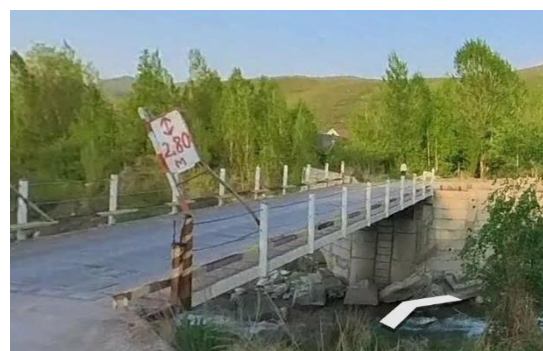
Figure 13: Bridge upstream of Kashka Su. (Google Streetview Image, Mai 2023)
