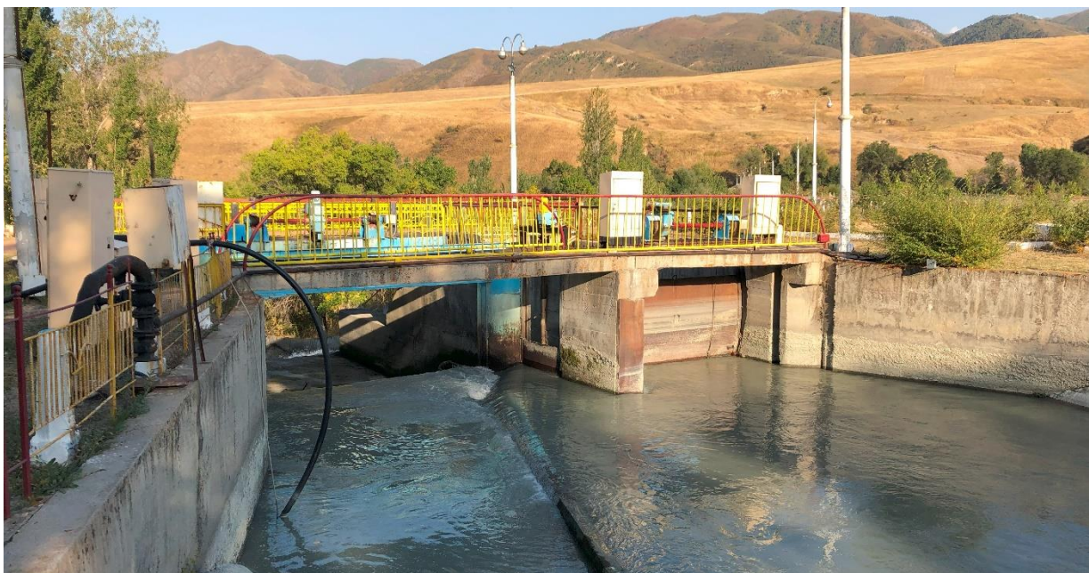
Figure 15: Dual gate opening of Kashka Su dam with overflow gate on the left and a radial gate to the right in direction of flow with ogee spillway crest in the back. (Image by Laura Niggli, August 2022).
