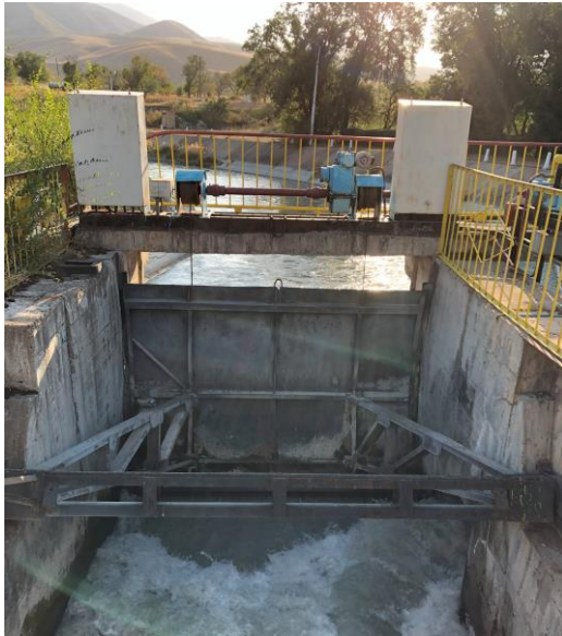
Figure 16: Radial gate design at Kashka Su dam. (Image by Laura Niggli, 2022)
