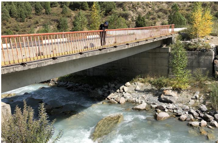
Figure 11: Access bridge to National Park. (Image by Laura Niggli, August 2022)
